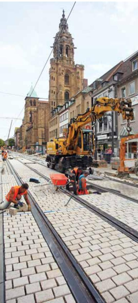
The international supplier of rail fastening systems Edilon Sedra presents the newly-developed trackbed structure Infundo-LR-MT at InnoTrans. The company claims that this system is specifically designed for heavily-used urban transport corridors, such as combined light rail and bus lanes or tram line sections which are shared with normal automobile traffic. The trackform has been developed following a suggestion by Heilbronn's municipal authority.
